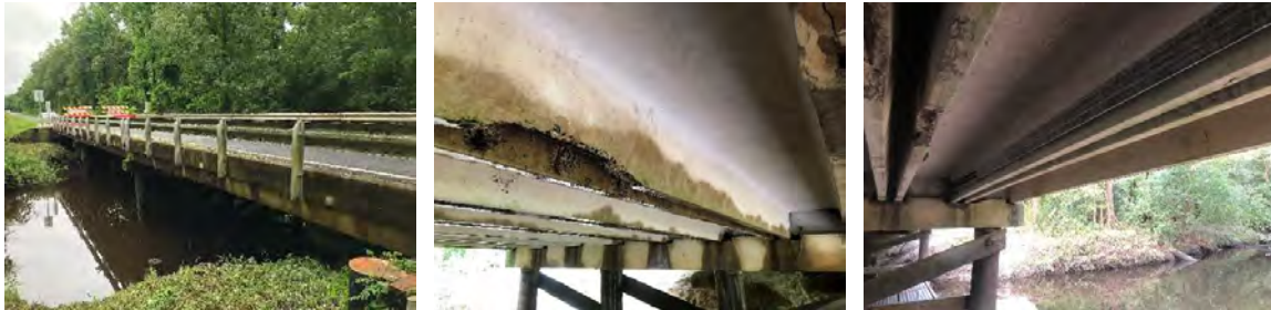
Figure: Deteriorated PC bridge retrofit using prestressed MF-FRP system.
