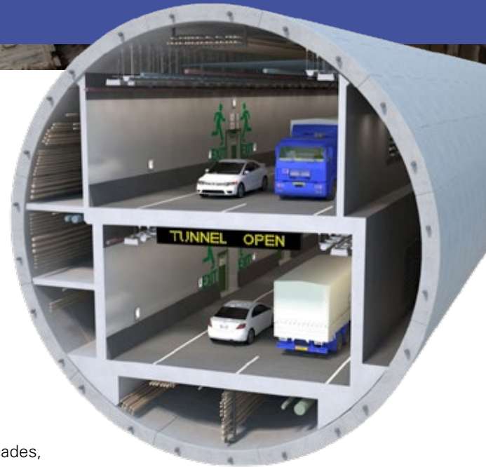
The tunnel has two levels of traffic. (Graphic courtesy of Yang Jiang)
