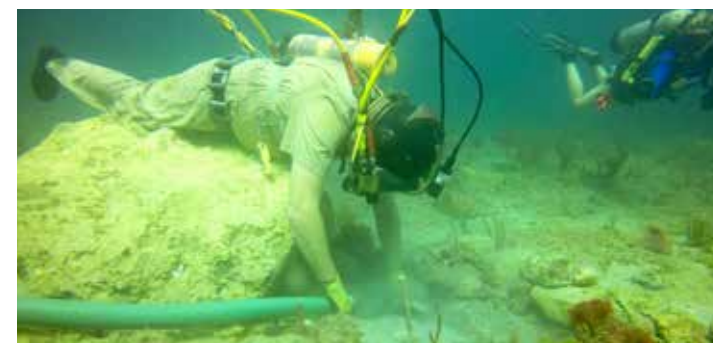
Loose rubble was removed, boulders placed and underwater cement used to create a stable structure.
