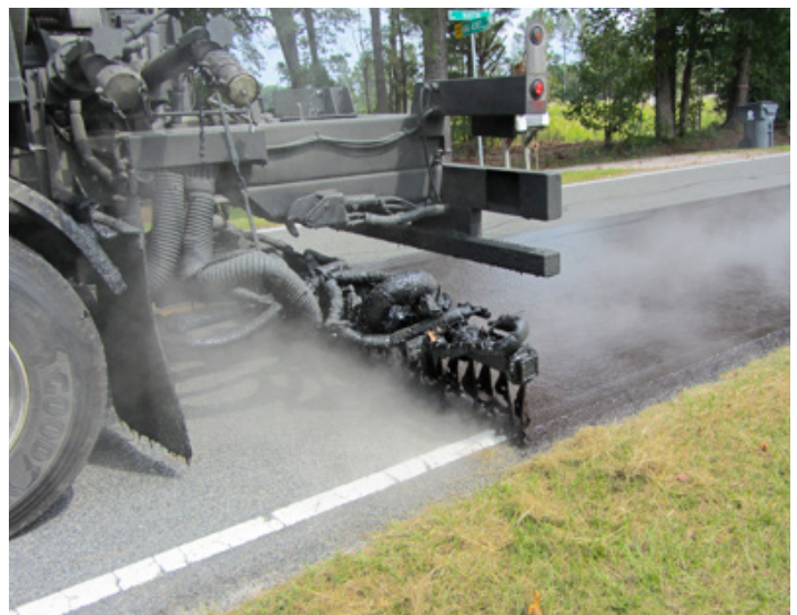
Spraying a tack coat on a North Carolina roadway. Image by R. Kim.
