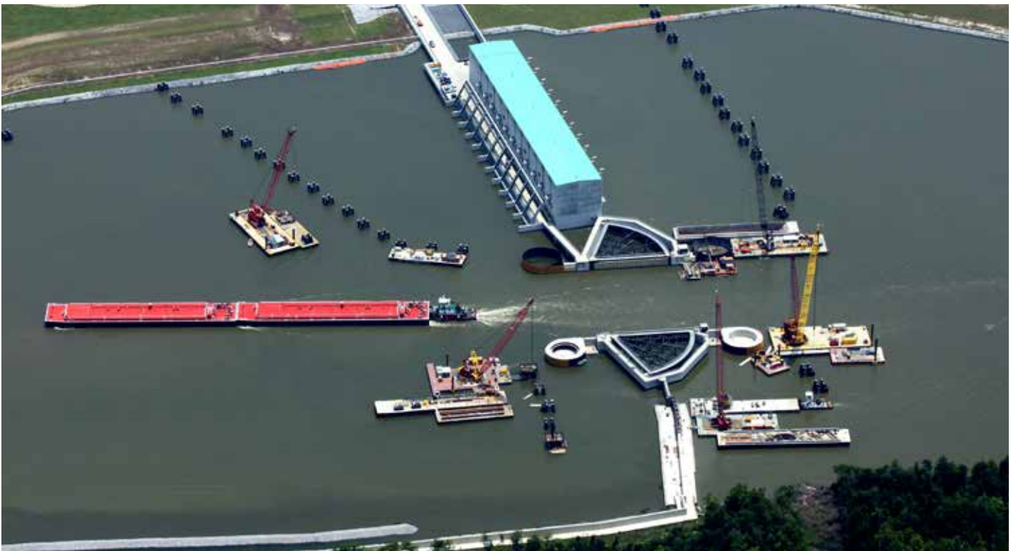
Cranes finishing work on the Gulf Intracoastal Waterway West Closure Complex, which reduces the flooding risk to communities on the west and south sides of New Orleans. The construction of the pump station and floodgates was the focus of the Zia Lecture in September.
