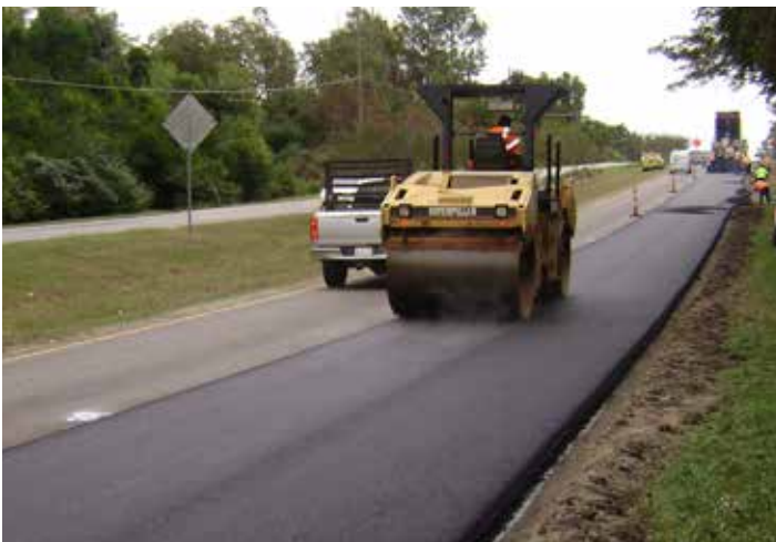
Asphalt paving compaction.
