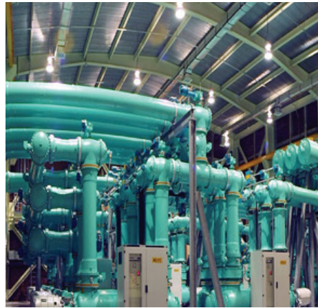
Gas insulated switchyard
