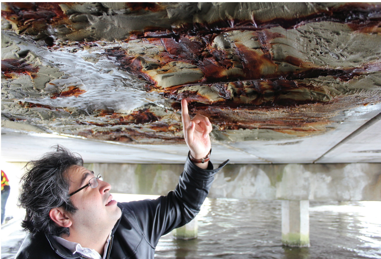
Dr. Pour-Ghaz examines the deteriorated bridge slabs
