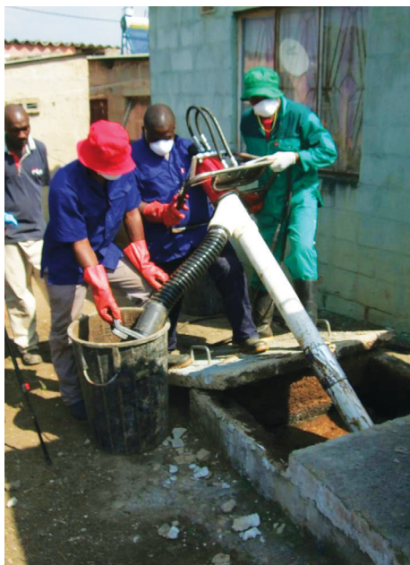
Pit emptying auger being used in Durban, South Africa
