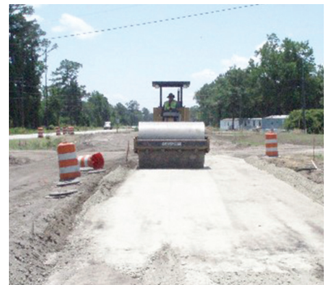
Compaction of the stabilization layer at the finished grade
