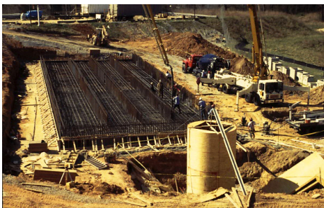
CFL structures lab lower mat and geotechnical sand pit.
