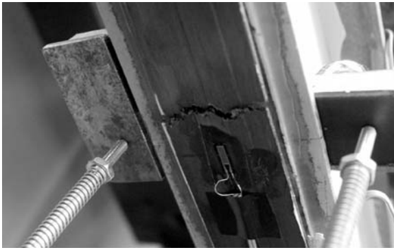
Figure 9 Rupture of CFRP strip for development length specimen using SP Spabond 345 adhesive and 203 mm development length
