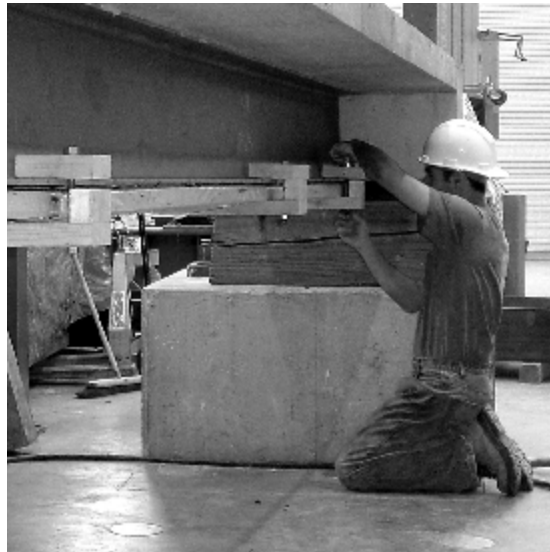
Figure 5 Clamping the HM strips within the pot-life of the adhesive
