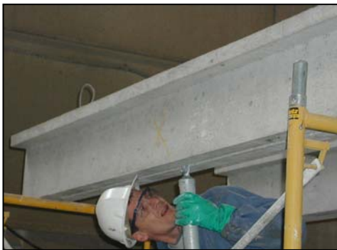
ii-filling the groove with epoxy
