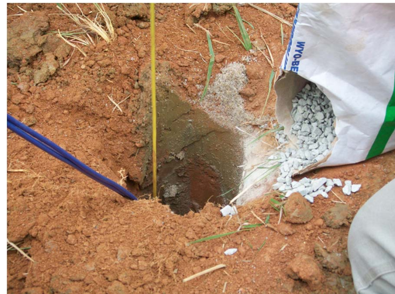
Filling with Bentonite
