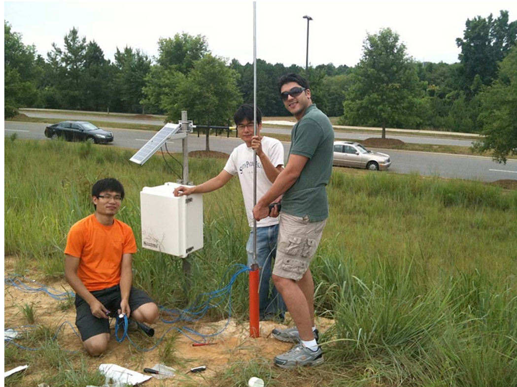
Installation of in-place piezometer
